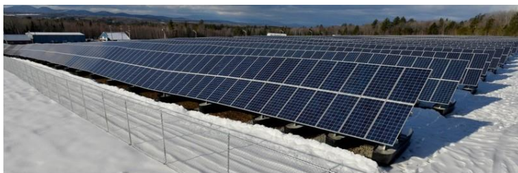
The Madison Electric Works solar farm consists of about 26,000 panels and occupies nearly 22 acres in the Madison Business Gateway. The project, which cost $10 million to install, is expected to produce about 5 megawatts of power. Michael G. Seamans/Morning Sentinel
